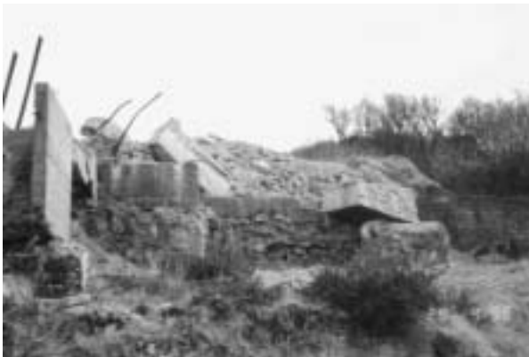
Figure 2: Remains of stone bases with loose blocks and dangerous metal work, Holman's Quarry (c. Kerrier District Council)
